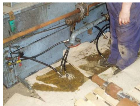
Spill mats in use
